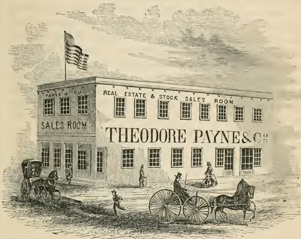
Formerly the Jackson House, south-west corner of California and Montgomery streets.
